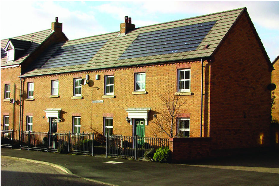
Housing with roof tile photovoltaic systems at Newcastle Great Park
