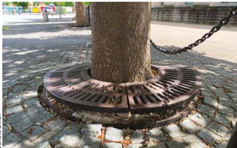
Constrained planting conditions exposing the tree roots and leading to pavement lifting (left), and (right) a tree that has outgrown its tree guard
