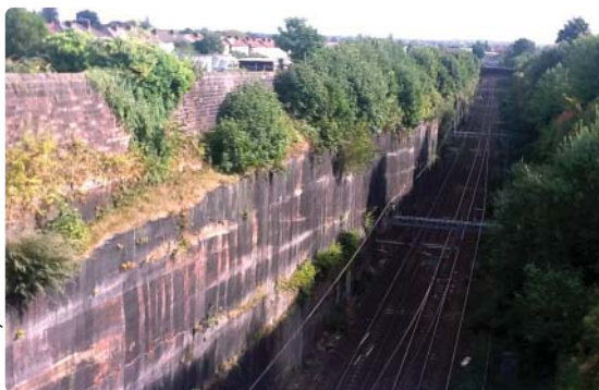
Olive Mount cutting—excavated by hand, with a little help from gunpowder; subsequently widened and recently electrified
