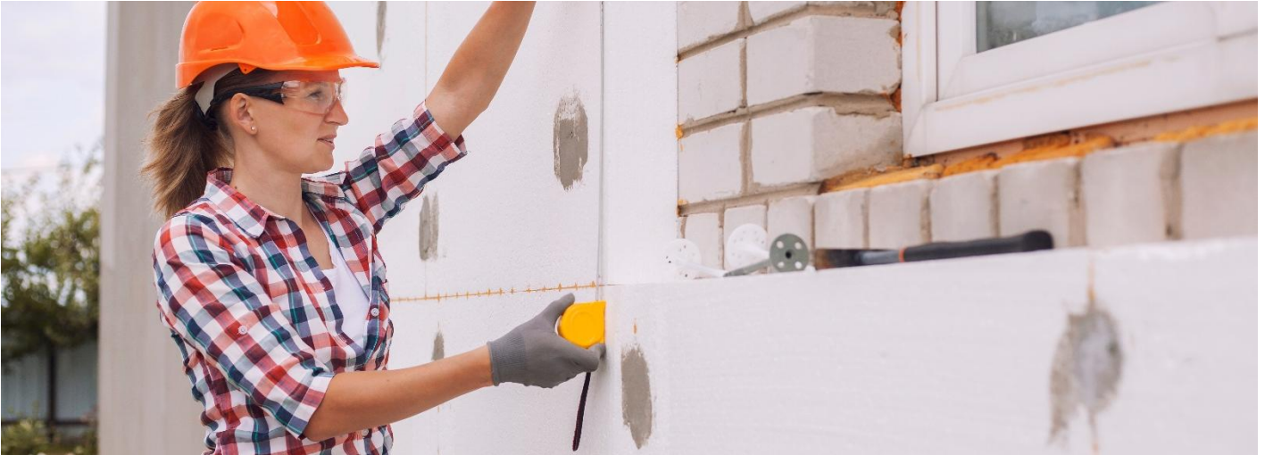
Figure 1: External insulation being fitted to a property façade. Source: Titov Dmitriy / Shutterstock.com
