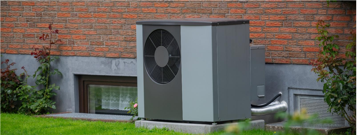
Figure 2: An air source heat pump installed outside a building. Source: Snapshot Freddy / Shutterstock.com
