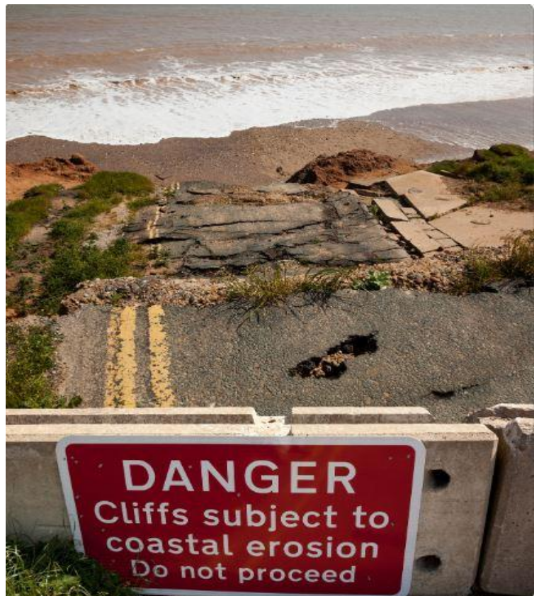
Figure 1: A road that has collapsed due to cliff fall. Source: Gabby Jeffs / TCPA.
