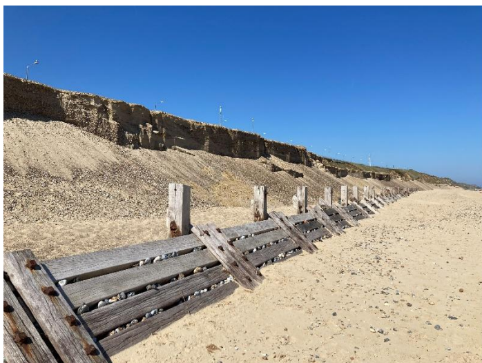
Figure 3: Wooden breakers on the coast in North Norfolk. Source: TCPA
