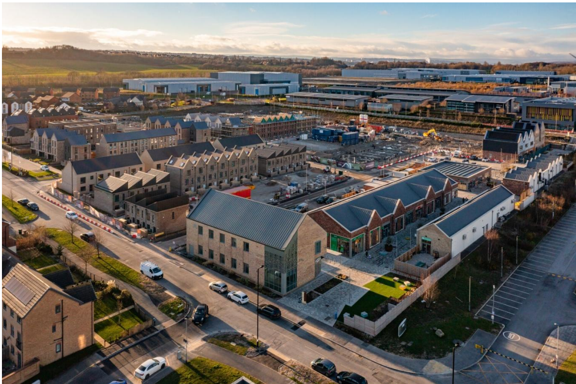
Olive Lane is being delivered as part of a new town centre at Waverley in Rotherham. The project is a case study in the guide on delivery by a master developer.
